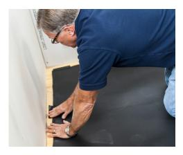
Lay out the pad material and cut it to fit with a gap of 1 inch between the pad and the wall. At the wall with the thermostat, leave a gap of 2 inches to act as a channel for the wires to run in.
