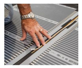
This sensor prevents the floor from overheating.
