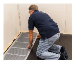
Remove shoes and work in stocking feet when installing film. Be careful not to drop objects on the film.
