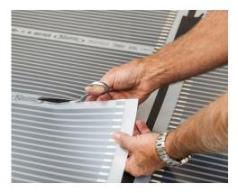
In some cases it may be necessary to trim the length to fit. Film may be cut only in the  $1\frac{1}{4}$ -inch clear areas between the carbon heating elements.
