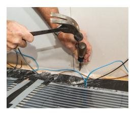
Use a hammer and chisel to cut a notch in the drywall and wall base plate so that there is room for wires to go from the floor to the thermostat.
