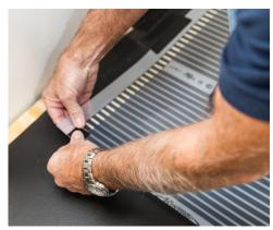
In the same way, use the mastic tape to cover all of the bare ends of each copper strip that do not have wire connections.
