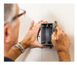
Place it on the wall about 5 feet above the floor. Make sure that it is not near any other heat sources and is out of direct sunlight.
