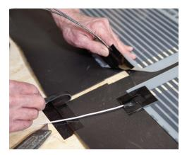
Channels for the wires and connectors must be cut in the underlayment mat. Use a utility knife to cut the channels, place wires into channels, and cover the channels with duct tape.
