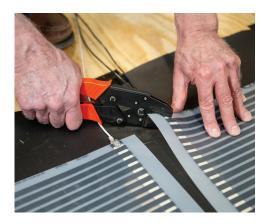
Run the other end of the wire to the corresponding corner on the next film panel to the right—allow a little slack. Shorten the wire if necessary and strip the end. Also strip the insulation from the end of another piece of black wire. Crimp both wires into a connector clip and crimp the flat end of the clip to the copper strip on the left corner.
