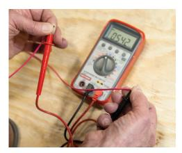
When all of the wires have been attached to the film, check the total resistance (ohms) to be sure that the connections are tight and that there is no damage to the film. Touch the ohmmeter leads to the 12 gauge wires that will go from the film to the thermostat and record the reading.
