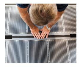
Film panels may be butted together or have some space between them depending on the layout of the room—they should never overlap! Use duct tape to fasten the film panels to the pad and/or to each other.
