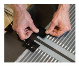
Cut 2-inch-wide mastic insulating tape into 2-inch squares. Apply a square of tape to both the top and bottom side of each wire connection and press them together firmly to form a tight seal.
