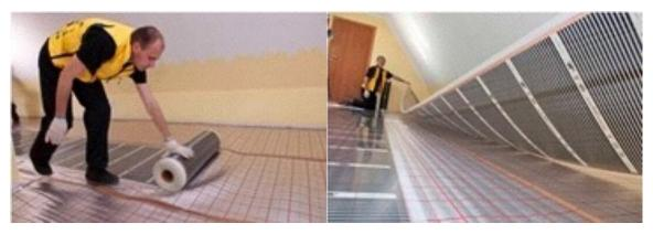
Cut out the heating film according to the scheme planned and put on the prepared surface, secure with adhesive tape. Each heating film line can be held in place by using a suitable adhesion tape such as duct tape along the ends and side of the film.
