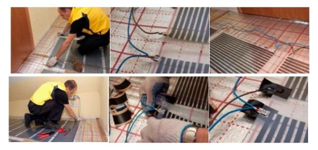
The connection ends and cold tails can be pressed into the underfloor insulation by scoring the underfloor insulation and firmly pressing the tails /ends into the scored underfloor insulation. It is advisable to tape over the connection tails and cold ends to keep the underfloor heating mats held in place during the instillation of your wood / laminate floor.
