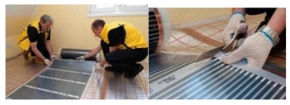
The heating film can be butted together but cannot be overlapped at any time.
