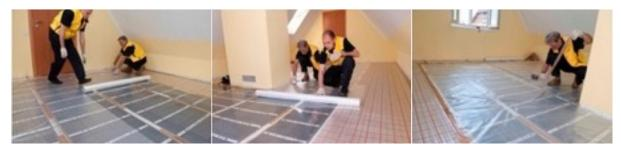
An electrical test of the adjusted heating film must be carried out by an electrician. All mats must be connected in parallel.
