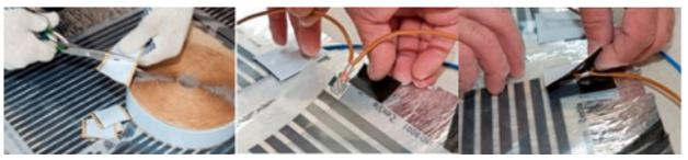
f) In the same way, use the mastic tape to cover all of the bare ends of each copper strip that do not have wire connections.
